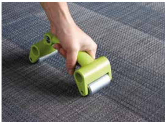
Smooth down the joints using the small seam
