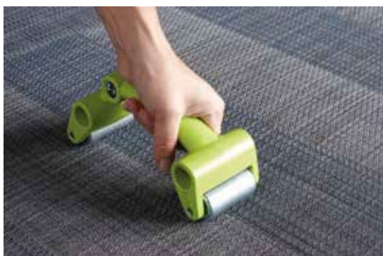
Smooth down the joints using the small seam
